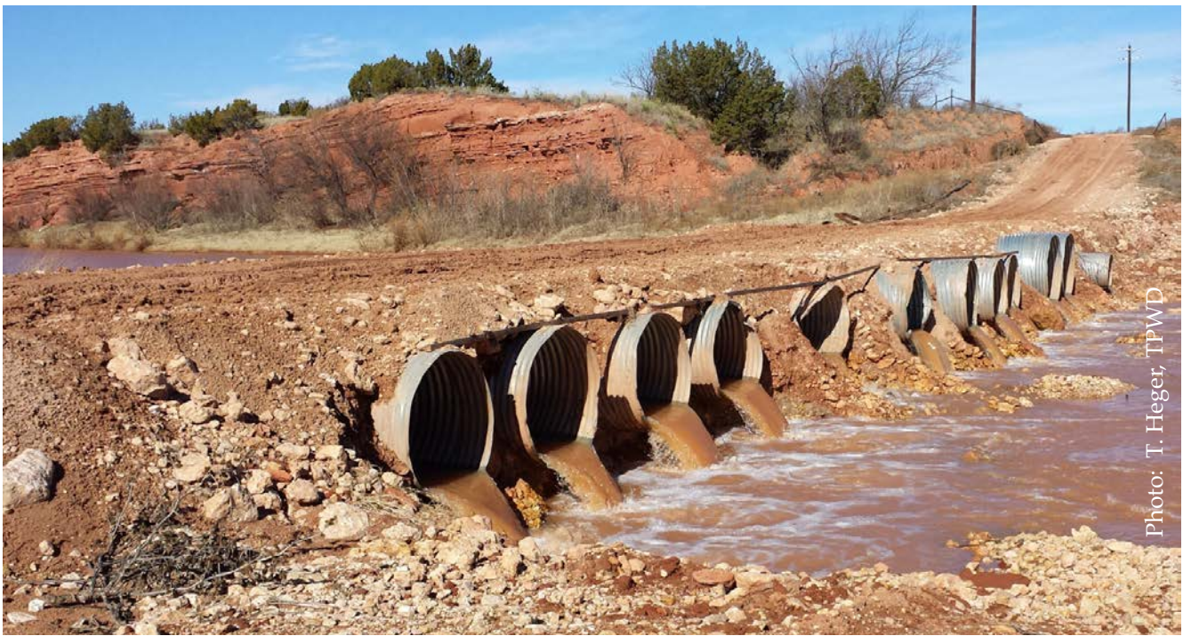
Figure 23 - Culverted crossing removed from the Double Mountain Fork Brazos River located in the Upper Brazos River Native Fish Conservation Area.
