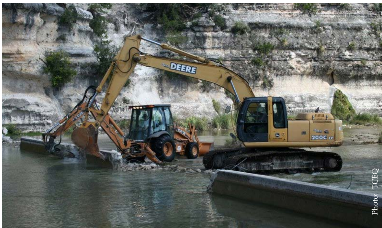
Figure 22 - Dam being removed from the North Fork Guadalupe River located in the Southern Edwards Plateau Rivers Native Fish Conservation Area.
