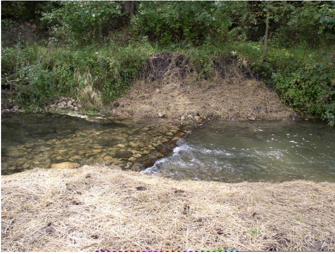
Fig. 13. Crosslog used to create pool habitat as part of a stream restoration project.
