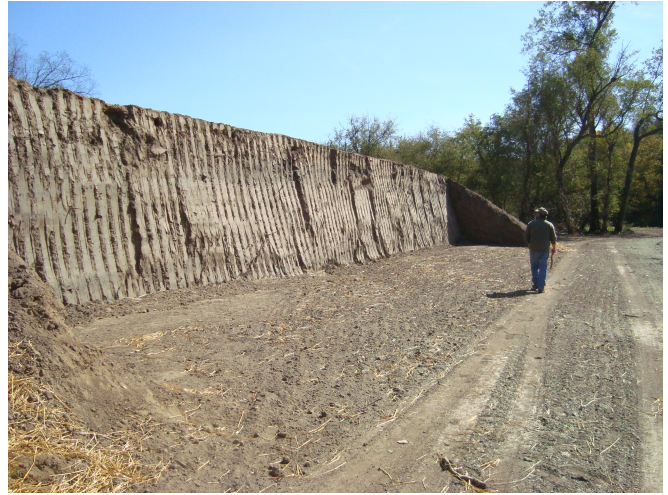
Fig. 10. Recently completed vertical nesting bank constructed as part of a stream restoration project.
