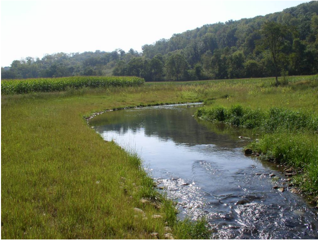
Fig. 4. Recently restored Driftless Area stream with stream buffer, sloped banks, and armored streambank toe.
