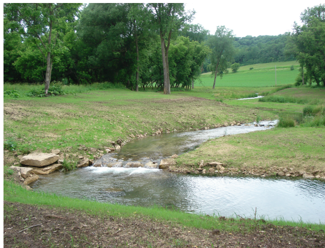
Fig. 1. Restored Driftless Area stream with armoring of the bank toe. Credit: Dauwalter.
