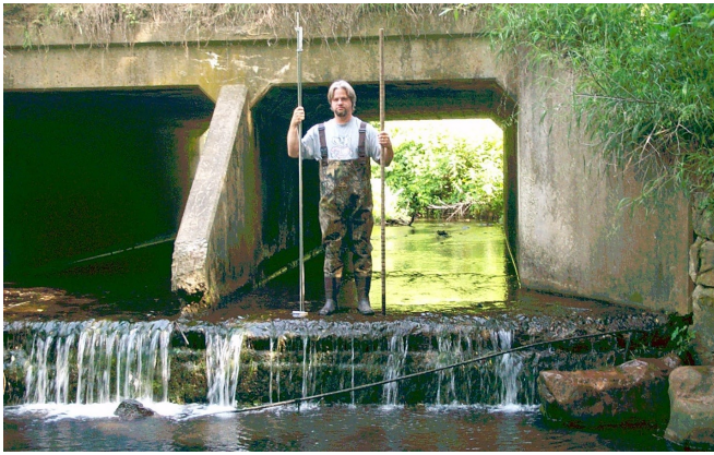
Fig. 14. Perched culverts, such as this culvert on Trout Brook in Dakota County, Minnesota, may prohibit trout movements during most stream flow conditions, except large floods. Credit: D. Dieterman.
