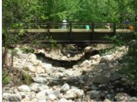
After – May 26, 2010 (looking upstream) 42' clear span; pre-manufactured steel bridge
