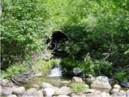
Before – July 20, 2006 (looking upstream) 6' diameter pipe; 3.4' drop
