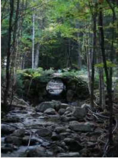
Before – September 22, 2008 (looking upstream) 6' diameter pipe; 1.2' drop
