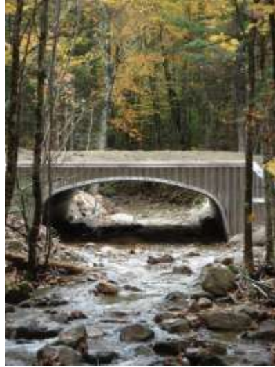
After – September 29, 2008 (looking upstream) 22' x 8' embedded aluminum box
