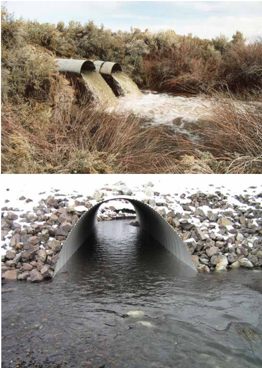
Figure 2. Culverts in Beaver Creek that prevented fish passage (top) were replaced with a fish-friendly structure in 2005 (bottom). Photos courtesy of Elko District BLM.
