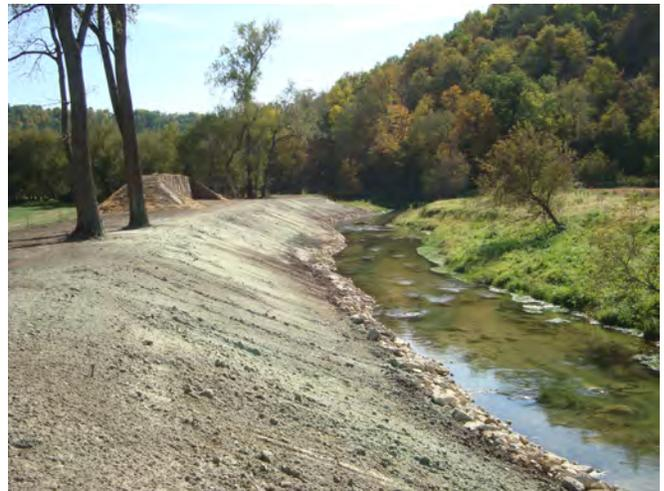
**Fig. 11.** Vertical nesting bank in background. Note its location set back from the stream channel.
