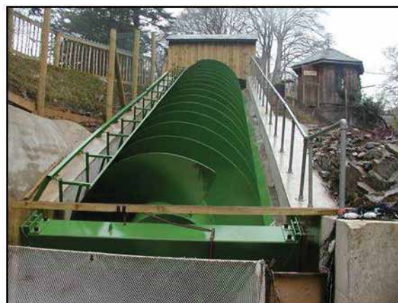
Figure 4. Archimedes screw turbine installed on the River Dart in the UK. Photo credit: Fishtek Consulting.
