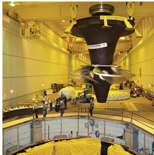
Figure 3. Voith Hydro Minimum Gap Runner (MGR) during installation at Wanapum Dam on the Columbia River in Washington State in 2005. Photo credit: Grant County Public Utility District.
