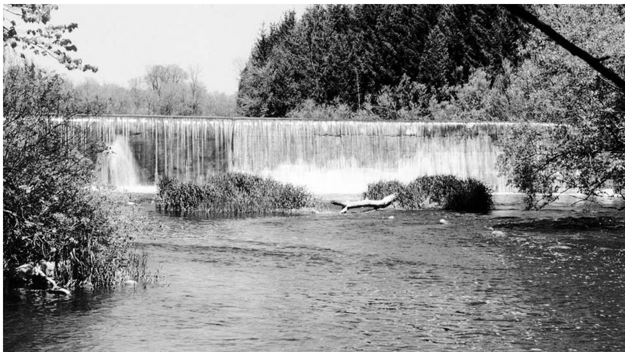
Franklin Dam on the Sheboygan River in Wisconsin. Photo: Edward Mueller.
