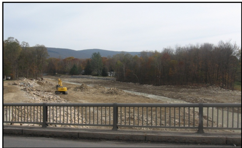
Figure 7: Construction of a new floodplain for the Roaring Branch, pre-Irene, above the Park Street Bridge in Bennington Vermont. (Kline, 2011)
