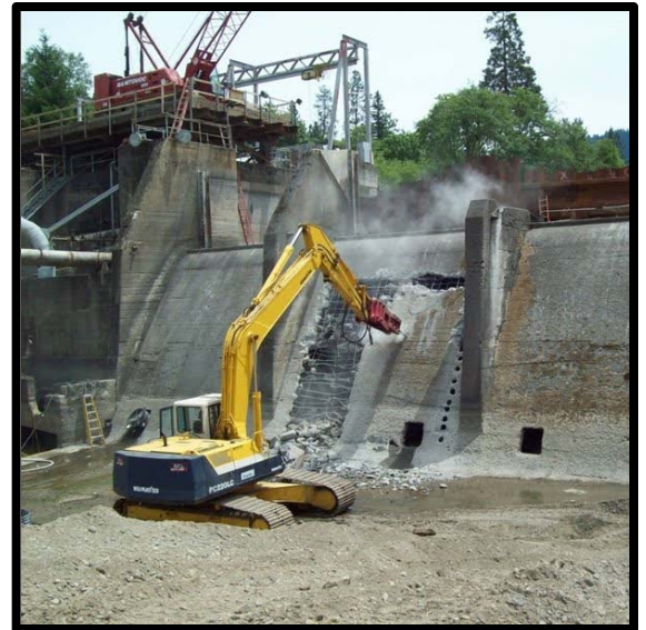
Savage Rapids Dam removal, Rogue River, Oregon
