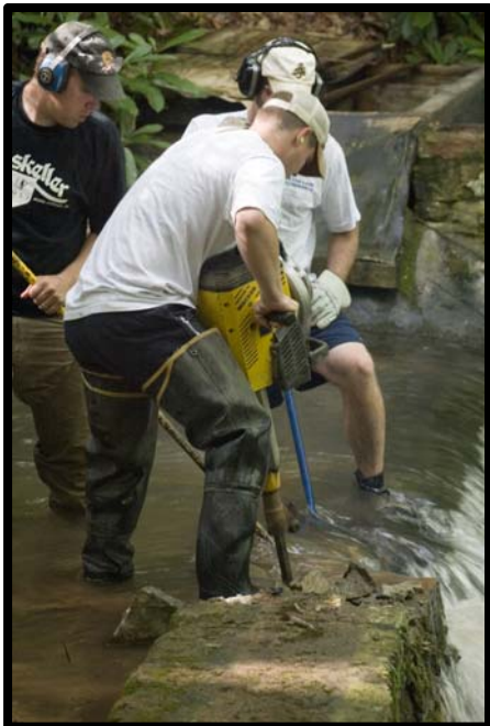
Bear Run Dam removal, Pennsylvania
