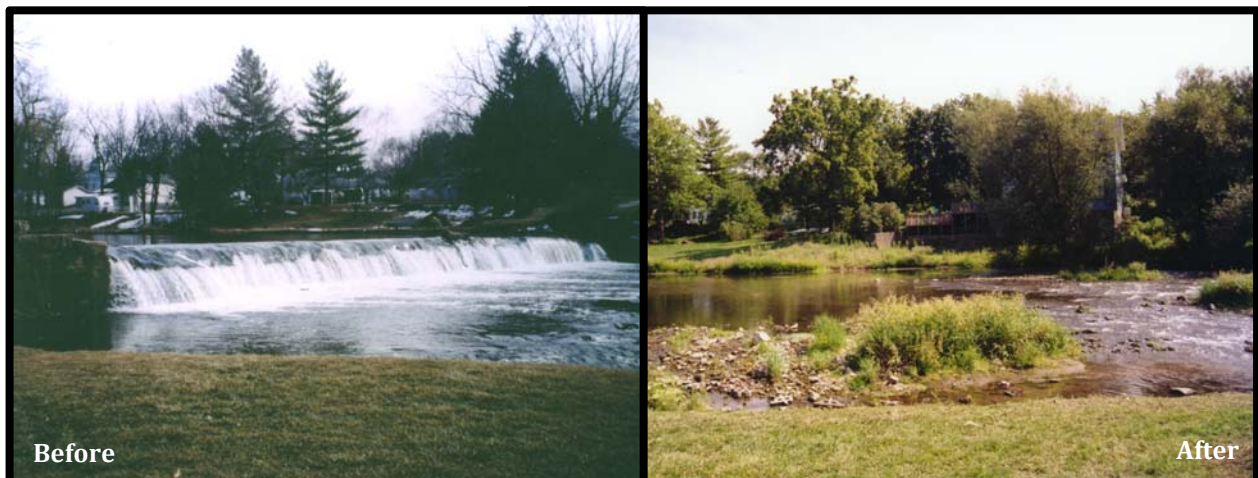
Shopiere Dam removal Turtle Creek, Wisconsin
