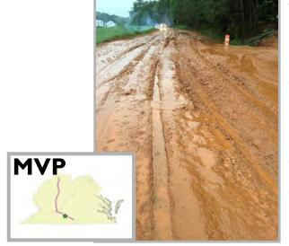
A Franklin County, VA hillside fails during construction of the pipeline covering Cahas Mountain Road in approximately a foot of mud and impacting nearby Little Creek. The failure occured on a 23% slope. Many segments of the ACP and MVP will traverse slopes of greater than 60%. Photo taken by volunteers with the Mountain Valley Watch.
