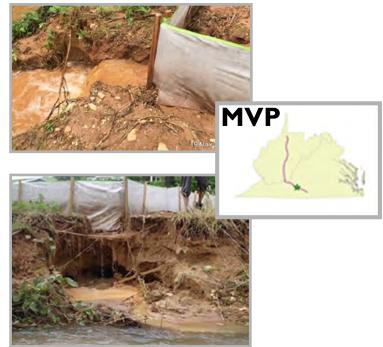
Concentrated runoff breaches a silt fence, erodes stream bank and enters Teels Creek in Franklin County, VA. Documented by Mountain Valley Watch volunteers along the pipeline.
