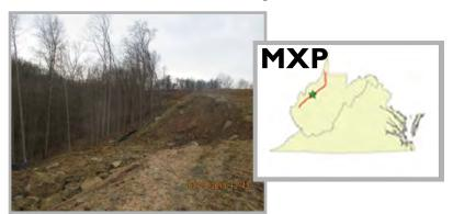
A major slip in Wirt County, WV on the pipeline route. Pipeline projects in the region, such as the Rover Pipeline, have continued to experience slips long after completion of the project.
