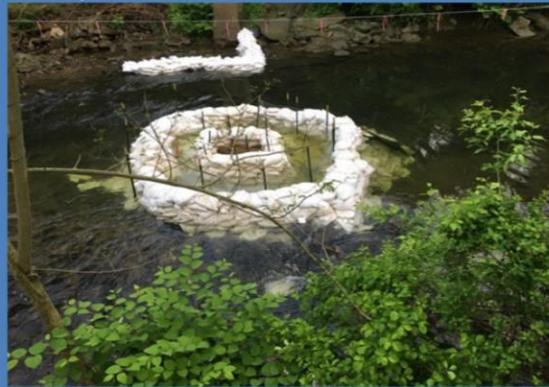
Sand bags used to contain leak of drilling fluid on Chester Creek in Brookhaven (Delaware County)
