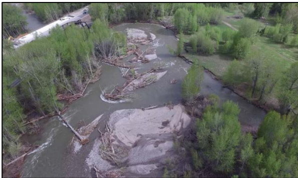
Figure 1. Aerial photo of the 'Bridge to Bridge' reach during the 2017 flood.
