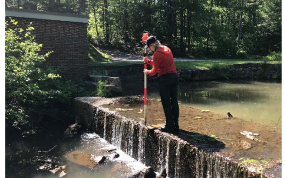
Frost Gully Dam; Max Daily Water Temps in impoundment are 3 degrees C higher than free-flowing reaches.
