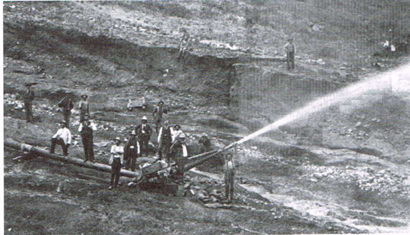
Hydraulic hoses at Gold Creek Mine. Source: Stanley W. Paher, Nevada Ghost Towns and Mining Camps (Berkeley: Howell North Books, 1970), 211.
