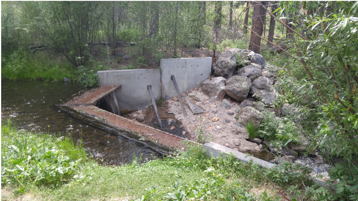
Figure 2. Fish passage barrier on the South Fork Little Colorado River, Arizona that protects an Apache Trout population from non-native trout downstream. These barriers are often designed to withstand certain flows and be effective for certain periods of time.
