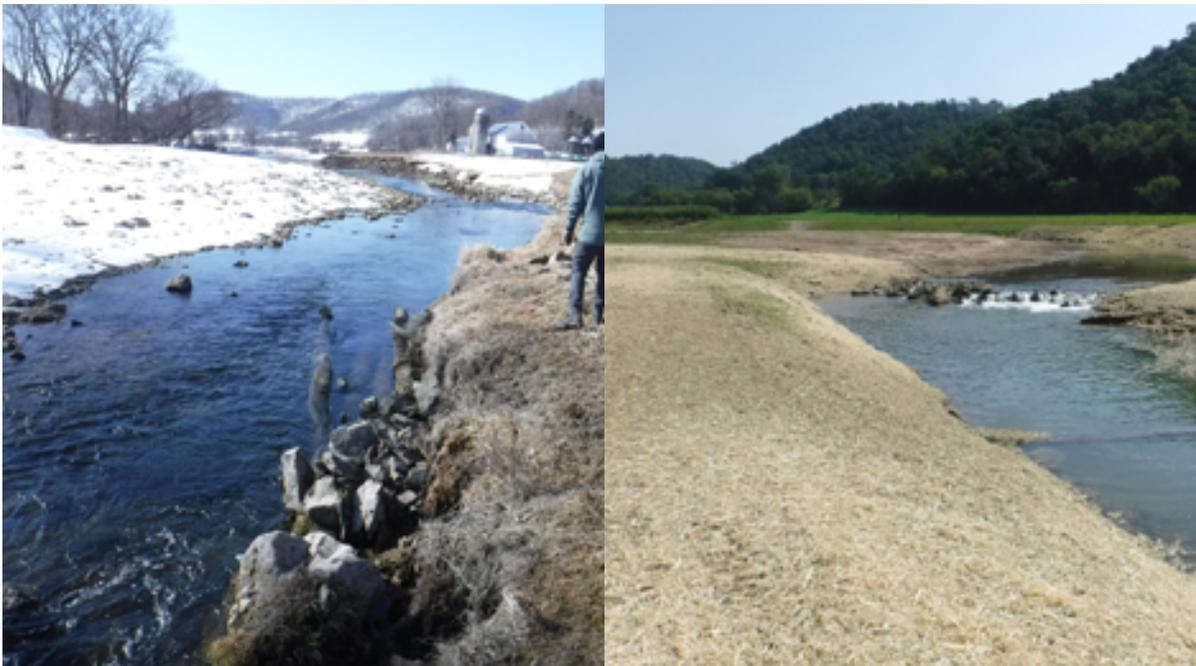
Streambanks throughout the 1.5-mile reach were stabilized with rock riprap. Trout habitat structures installed included rock weirs, bank logs, rootwads, and boulder clusters. The streambanks, as well as the floodplain, were regraded and seeded to grasses to reduce future flood damage.
