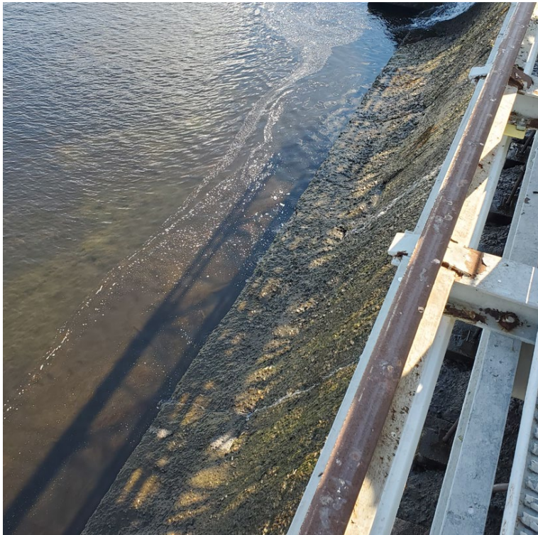
Figure 19. Deteriorated concrete along the spillway below the hinge boards at the Shawmut Dam.
