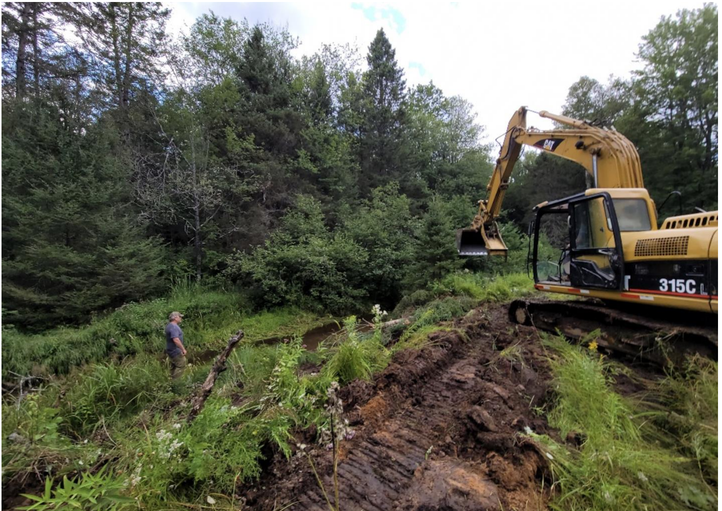
Local contractor Kanouse Outdoor Restoration overseeing woody habitat implementation
