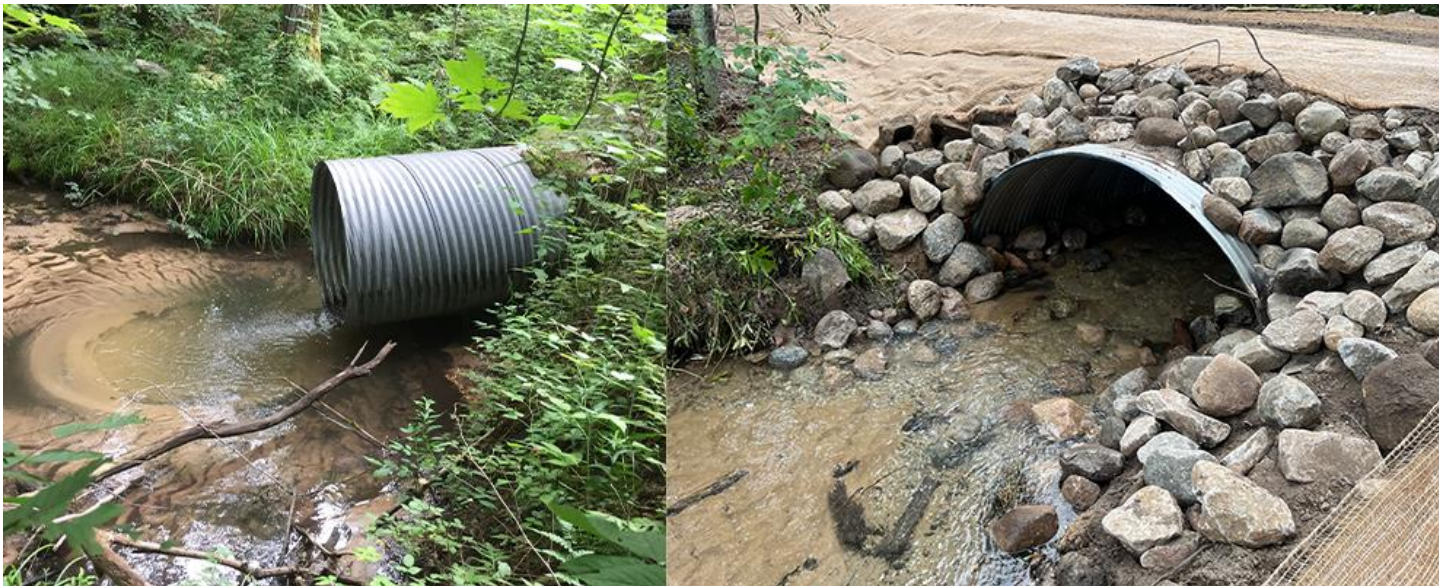
Before and After Photos of a culvert replacement on Peterson Creek
