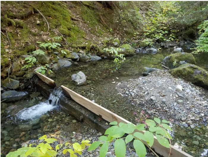
Figure 3. The current diversion that will be replaced with a fish friendly structure.
