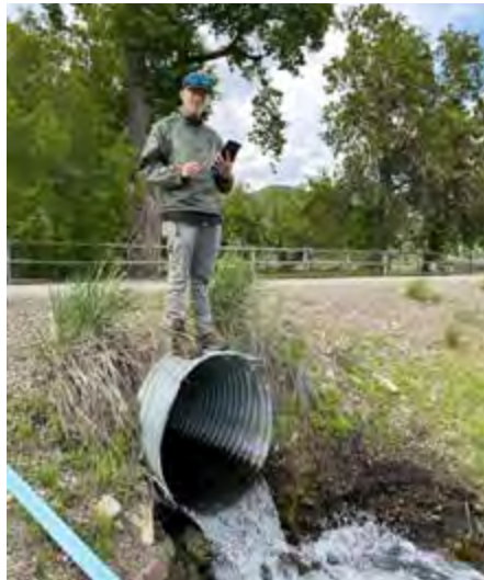
Carson Jones inventories a perched culvert in Idaho.
