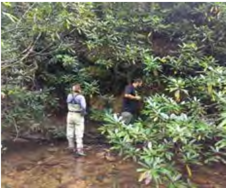
Bank stabilization on Kuykendall Creek.
