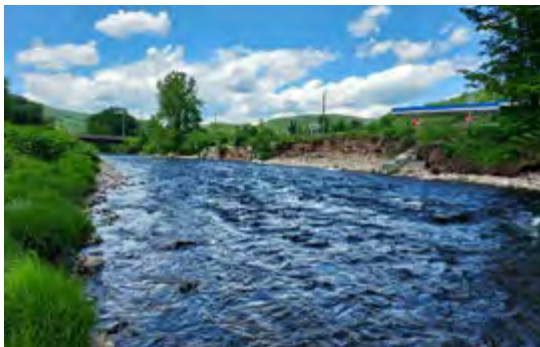
Erosive road bank in the Willowemoc Creek—a famous Catskill tributary that flows into the Beaverkill and eventually, the Delaware River.
