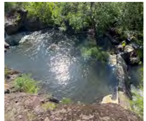
Small dam to be removed on Jenny Creek, a tributary to the Klamath River.
