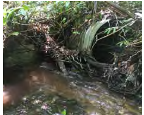
Culvert in the Cathy's Creek watershed.
