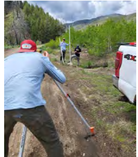
Sawyer Finley, Carson Jones, Owen Swavely survey a culvert in Idaho.
