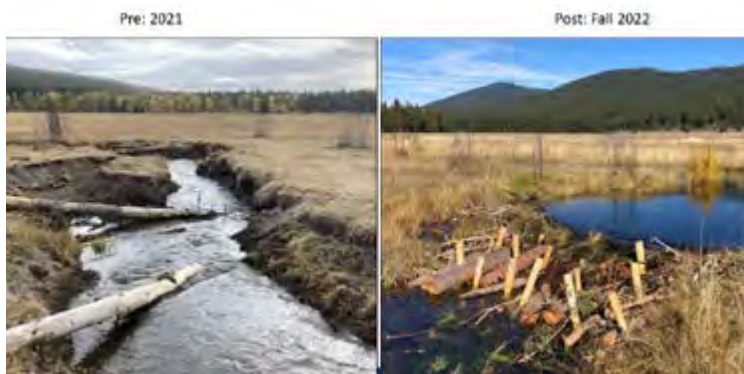
Implementation of process-based restoration on Sun Creek, Klamath Basin, Oregon.
