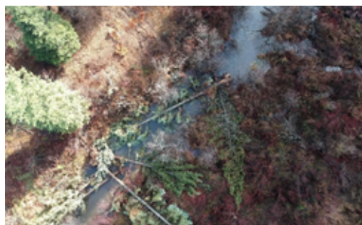
Newly installed log jam on East Fork Potlatch River
