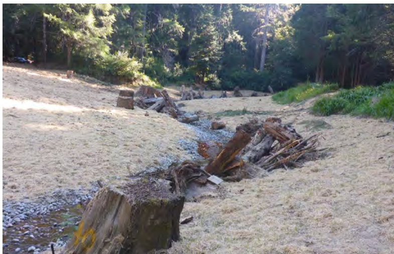
Large wood structure installed in the Jack of Hearts Creek
