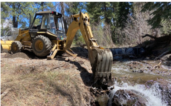
Constructing the Headache Creek barrier
