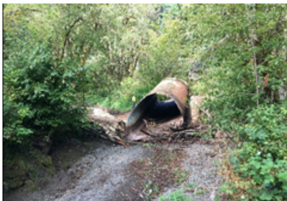
The above culvert removal and road decommissioning project reconnected Zeigler Creek in the Quinault River drainage. Note the person in a yellow jacket standing next to the culvert for scale.
