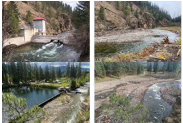
Photos taken before (left) and after dam removal (right)
