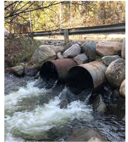
Lily River culvert project that received $300,000 from FEMA.
