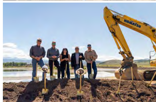
Breaking ground on the Colorado River Connectivity Channel Project in August 2022.
