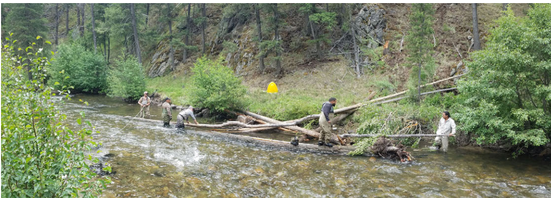
Figure 14—Large wood stream and floodplain habitat restoration on Panther Creek in the Salmon-Challis National Forest, ID, implemented in 2018 by Shoshone-Bannock Tribes, along with culvert replacements elsewhere in the watershed. Forest Service photo.
