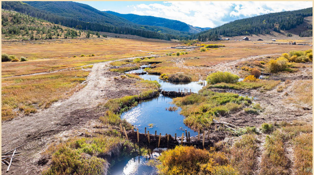
Figure 5—Beaver dam analogs (BDAs) constructed on Soda Creek, Dillon Ranger District, White River National Forest, funded through the Colorado Western Slope In-Lieu Fee Program. Courtesy photo by National Forest Foundation.
